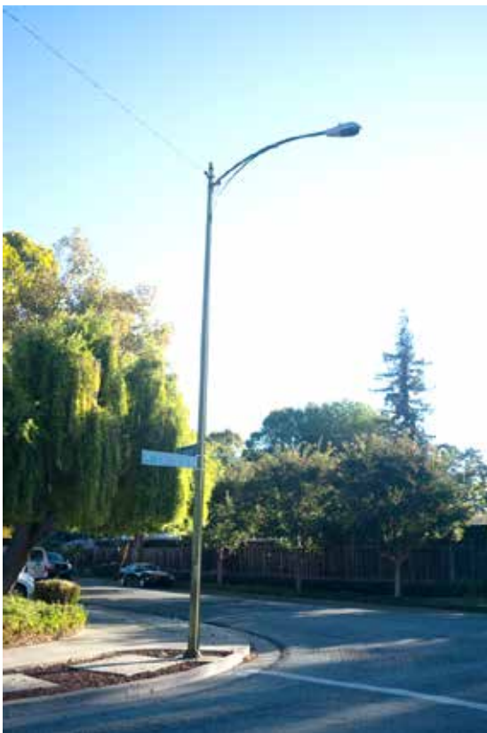
Fairglen Additions Santa Clara County, CA Photo 6 of 21 (Lightpost)
